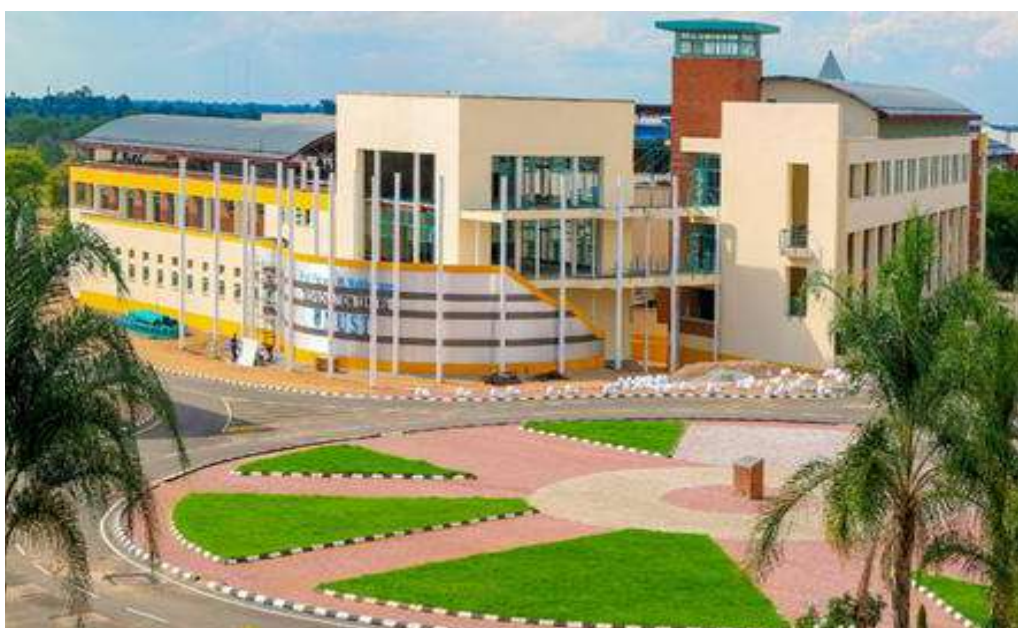
Technovation Centre at the National University of Science and Technology
