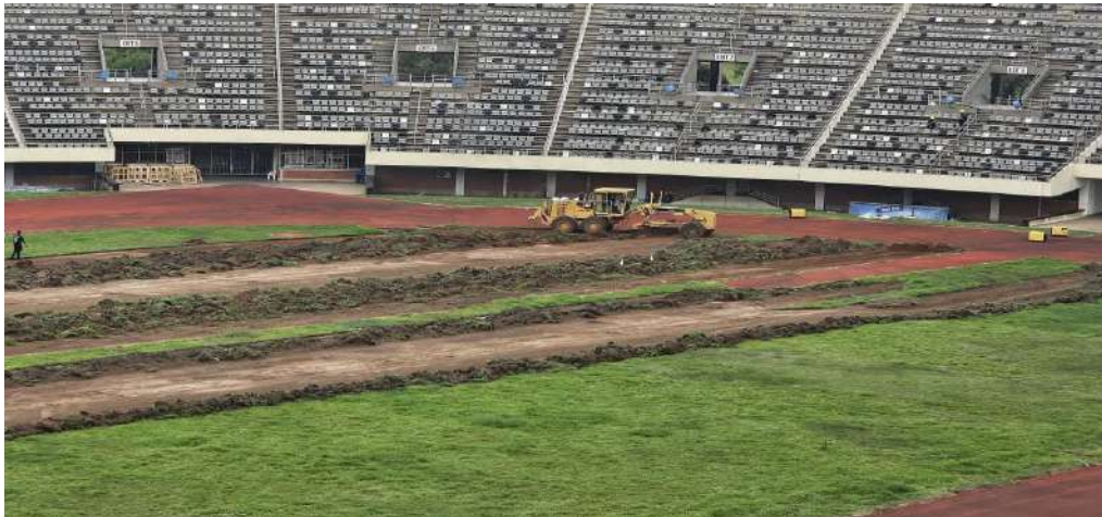
Bucket Seats Installation and Field Works
