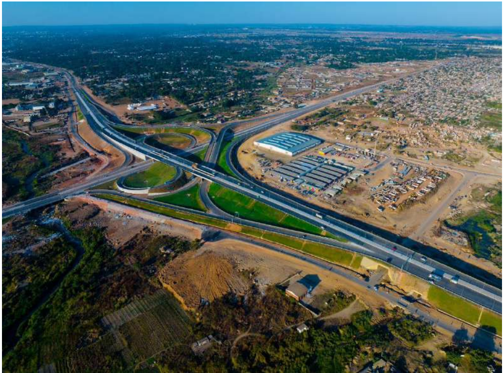
Commissioned Trabablas Interchange
