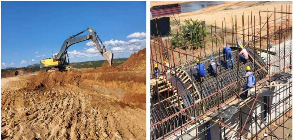
Construction of Kunzvi dam project
