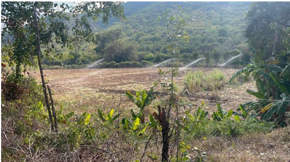
Mhakwe irrigation System testing, Manicaland
