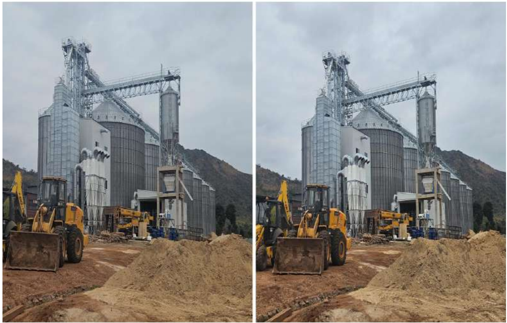
Mutare Smart Silos Under Construction
