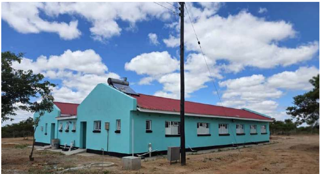
Bwoni Rural Health Centre Electrified
