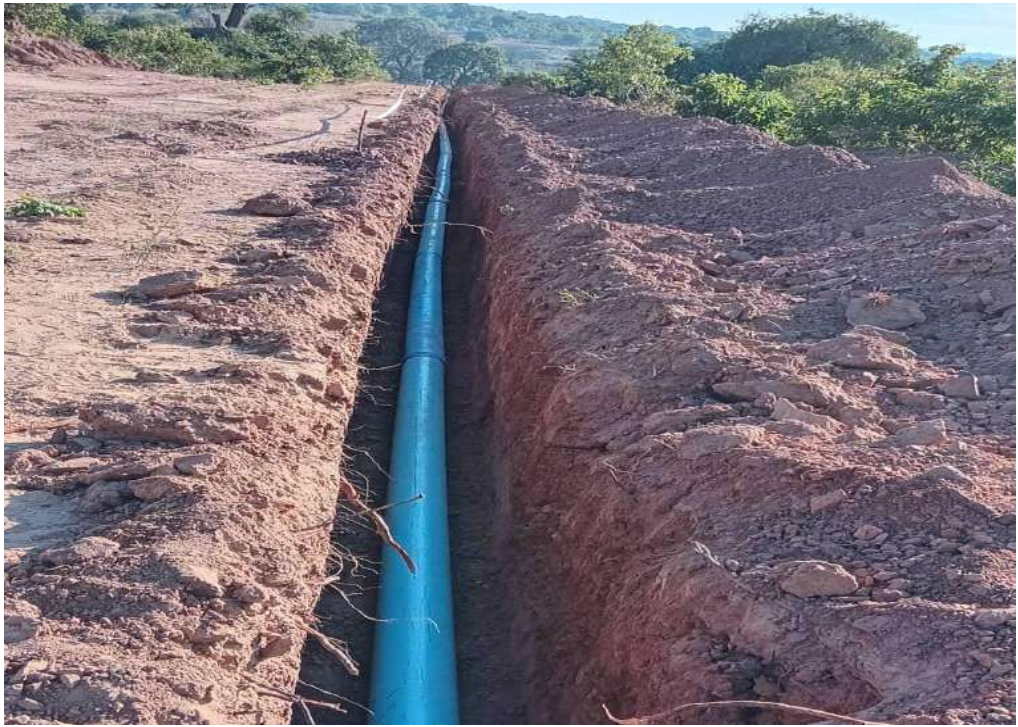
Musirizwi irrigation scheme pipe laying, Manicaland
