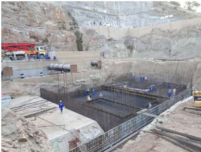
Reinforcement installation for 10MW Hydro powerplant foundation baseplates
