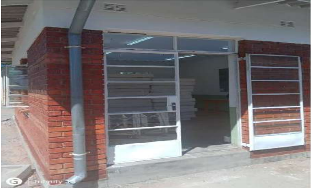
Renovated training school – Gokwe North Hospital
