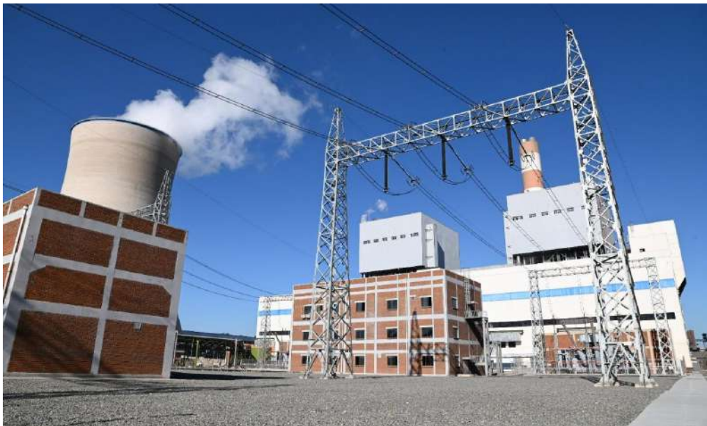
Hwange 7 and 8, Power Plant
