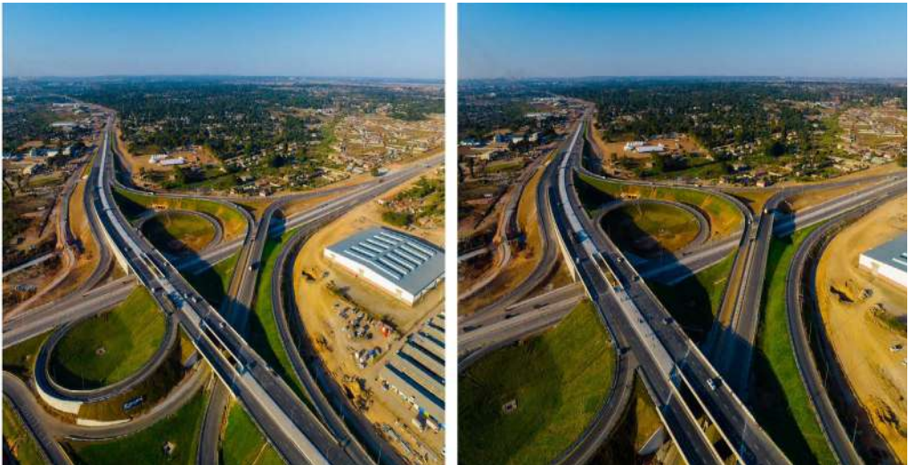
Commissioned Trabablas Interchange
