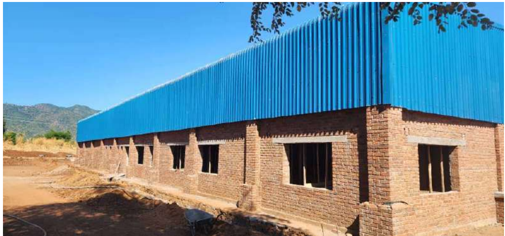
Completed Superstructure for the Muzarabani Masawu Value Addition Plant
