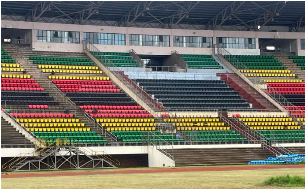
Installed Bucket Seats
