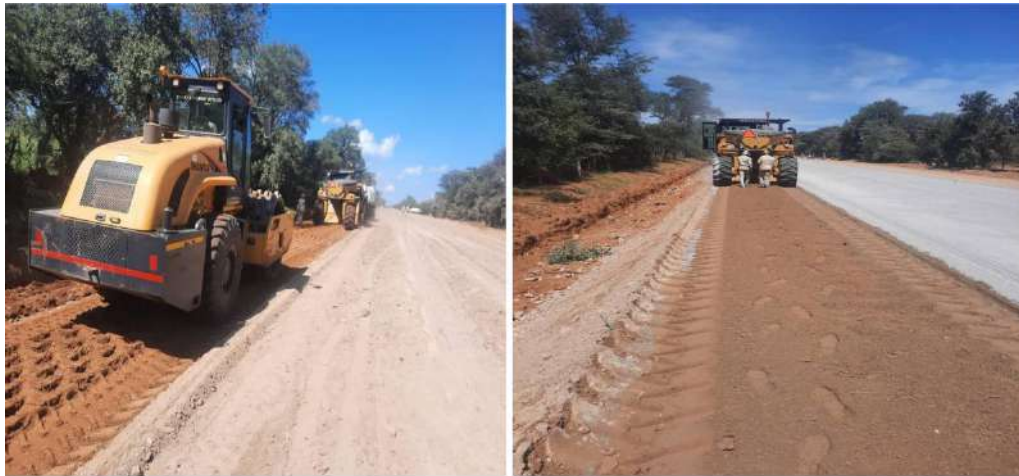
Stabilization of subbase on the Harare-Masvingo-Beitbridge Road - Mwenezi District Section
