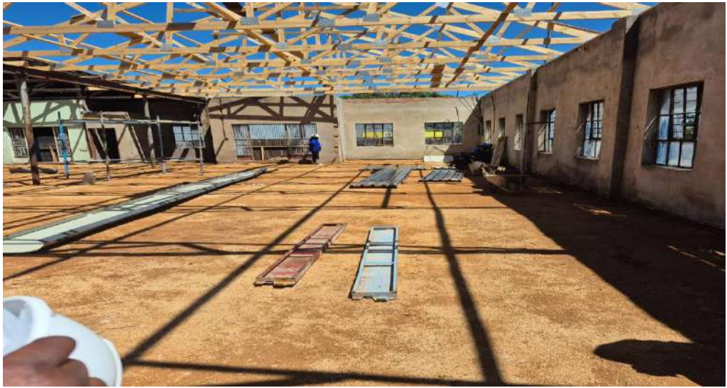
Bulawayo Textile Manufacturing Centre under construction
