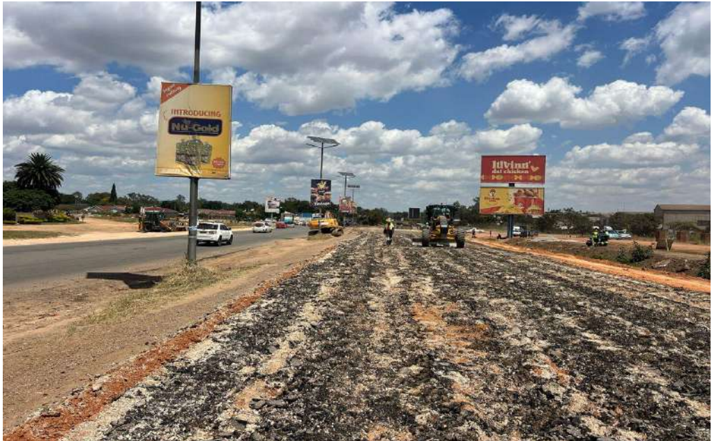
Ongoing Harare – Beitbridge Road Rehabilitation – Houghton Park Section
