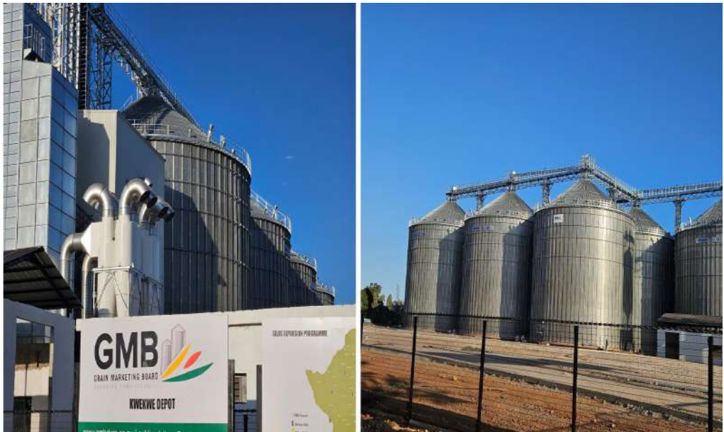
Commissioned Kwekwe GMB Smart Silo Facility
